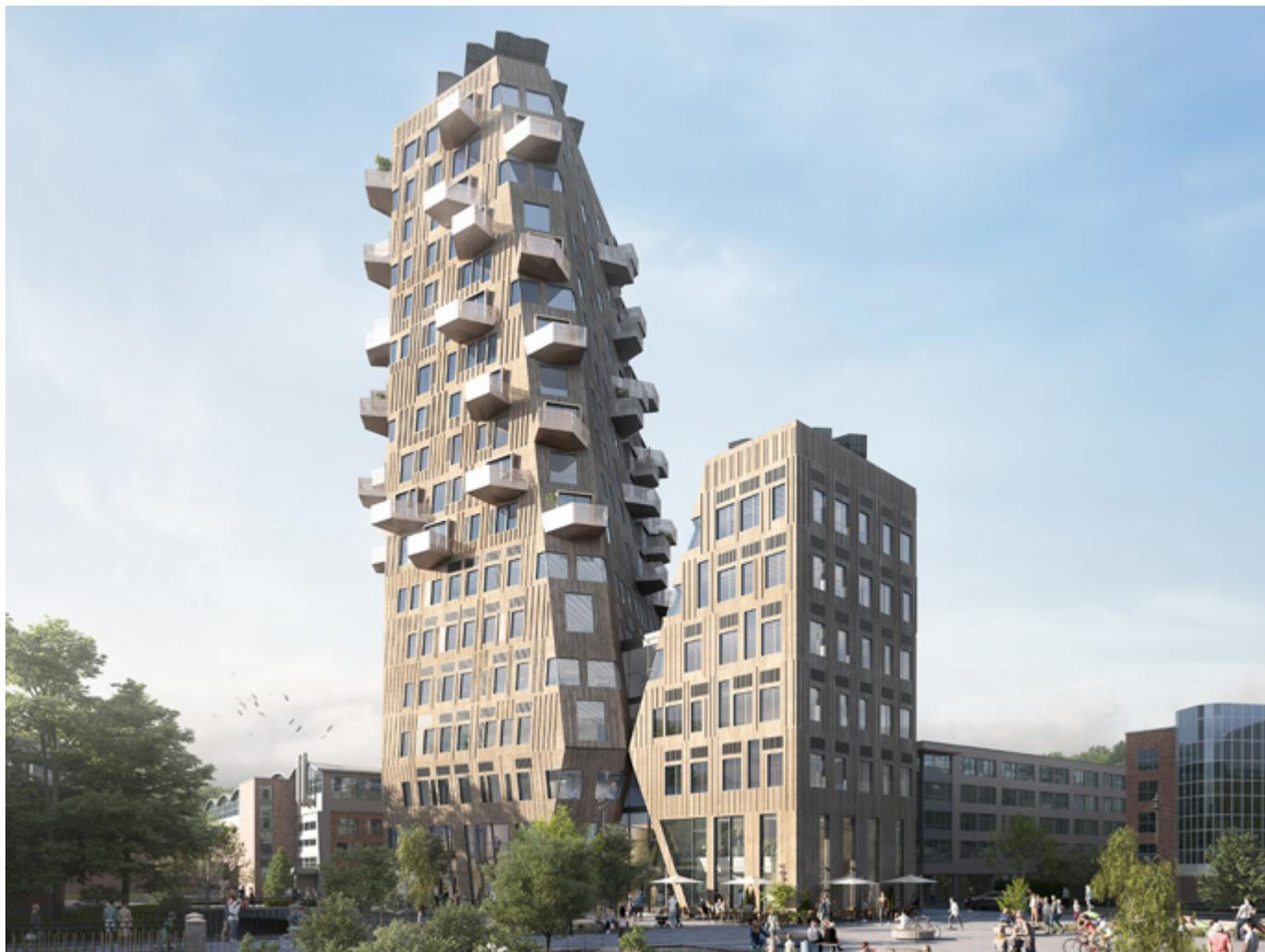
The newly built project is a 11,200 m<sup>2</sup> building at Gullhaug Torg 2A in Nydalen in Oslo, the capital of Norway. It is expected to emit 50% less CO<sub>2</sub> from materials, transport and energy compared to other comparable buildings, and purchase 0 kWh of energy for ventilation, heating and cooling.
